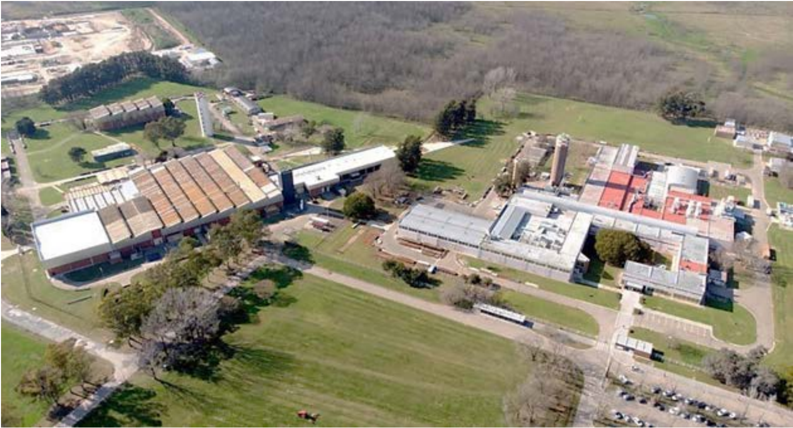
Headquarters and three tailored facilities to manufacture nuclear components and tubes.
