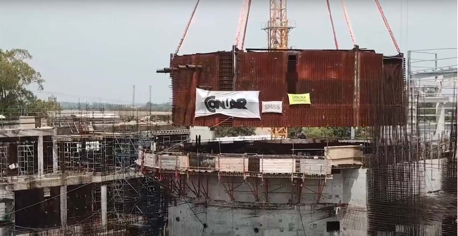
Manufacturing & Assembly of Module 10 from CAREM25 Liner Contention, see it at Youtube .
